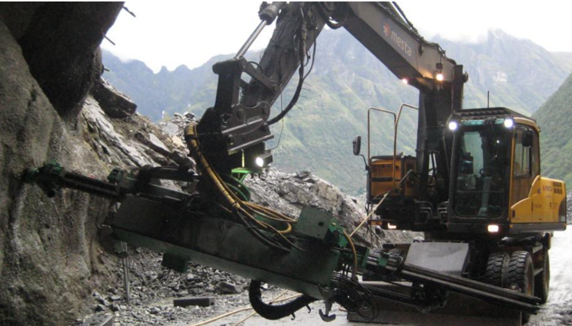
Ground Reinforcement – French Alps
