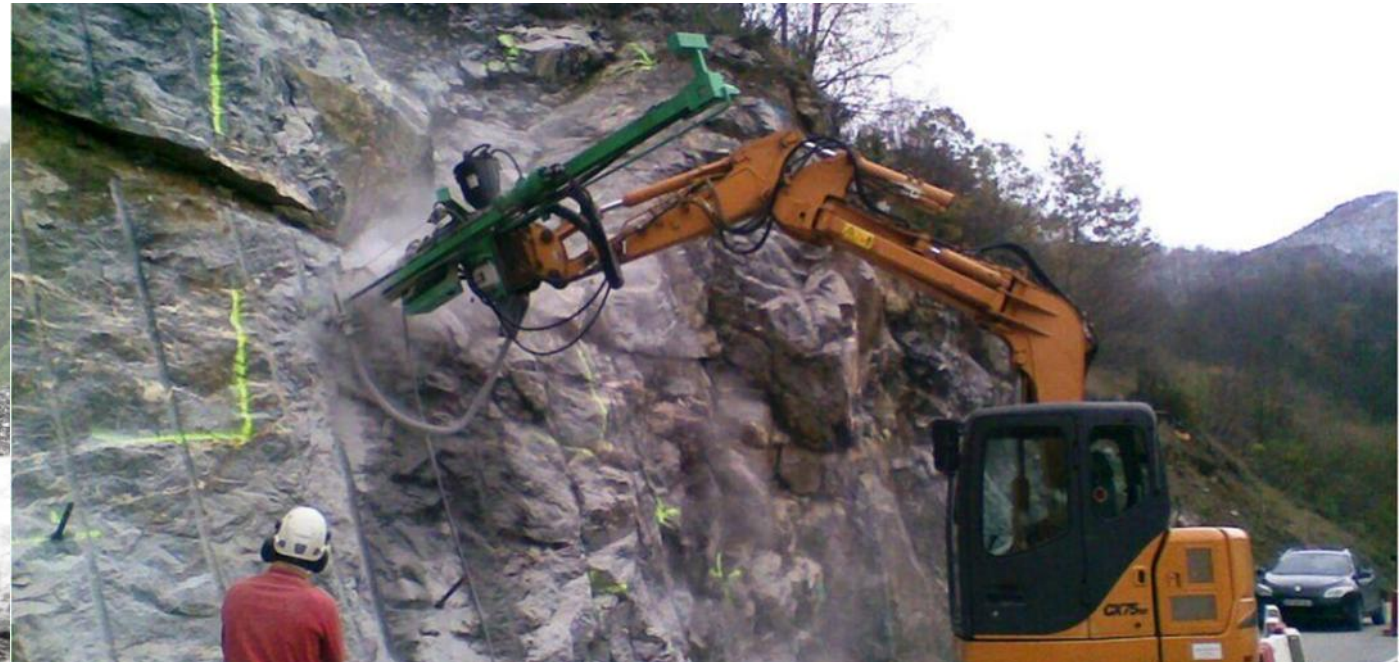
Ground Reinforcement – French Alps
